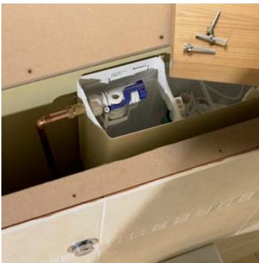
Access to the cistern via removable shelf.
